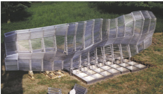
Manufactured sections delivered to site prior to construction.
