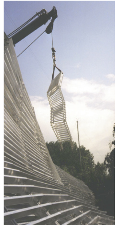
Sections lowered in place and assembled on pre-built foundations.
