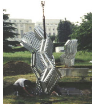
Sections lowered in place and assembled on pre-built foundations.
